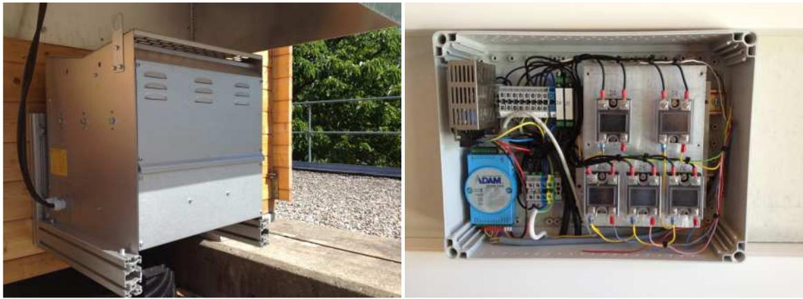
Figure 10: 2.5 kW programmable active load
