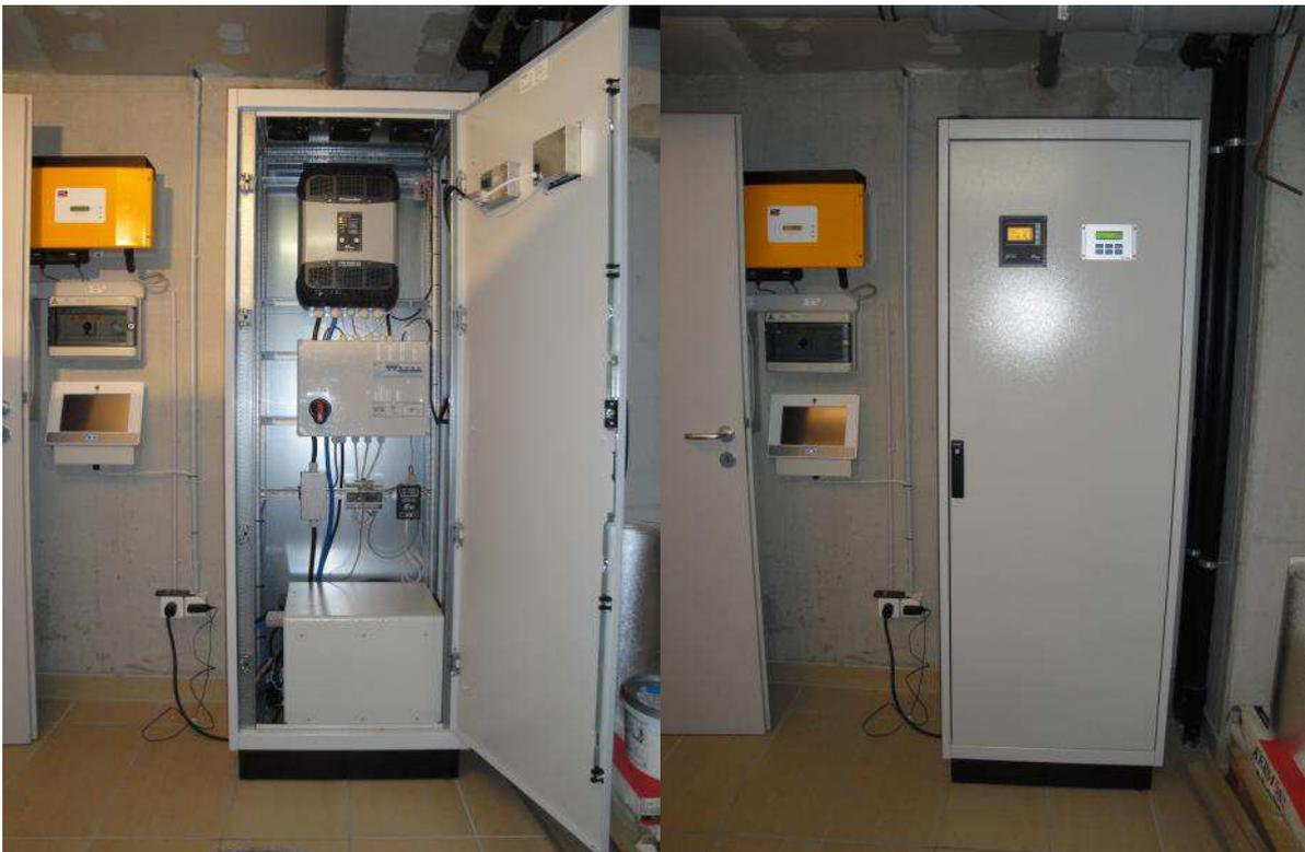
**Figure 7: Battery-to-grid system installed in the households**
