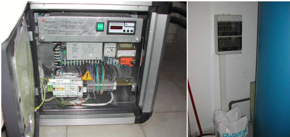
**Figure 8: Heat pump control panel and HAC installation**
