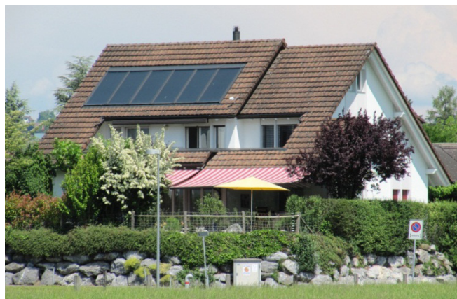
Figure 5.2: Single family home with 15 m 2 solar thermal collectors.
