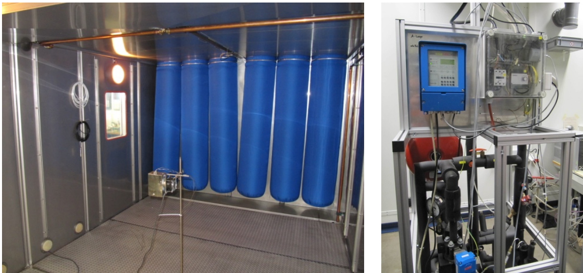
Figure 7.5: Climatic chamber for the outdoor unit of air source heat pumps (left) and emulation module for the ground heat source (right).
