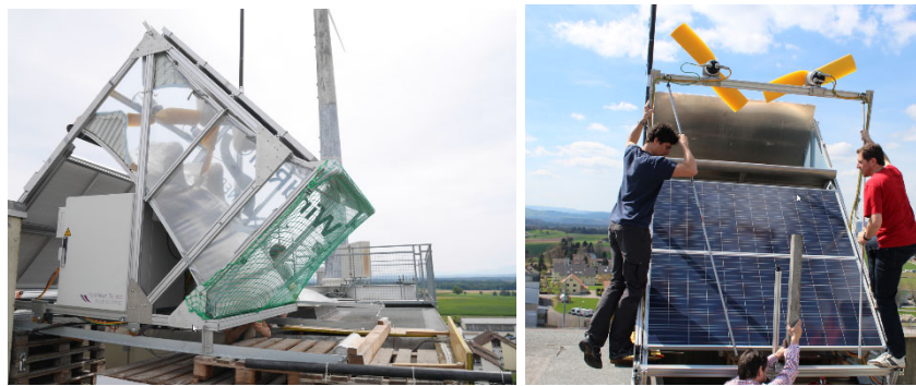
Figure 26: Rotor maintenance functionality and WindRail maintenance position
