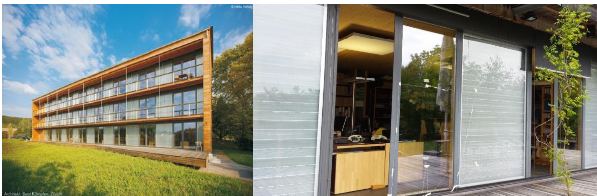
Figure 15: Marché International AG building and outside view of the measurement set-up; source: (Hellwig) left picture, (greenTEG, right picture)
