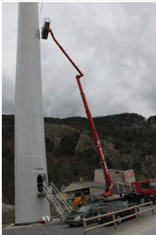
Installation at 31m height with man-lift
