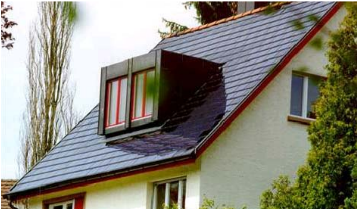
Photovoltaic roof in Vischer (Switzerland), 3 kW, 1998, built by Atlantis Solar Systems (Bern, Switzerland)
