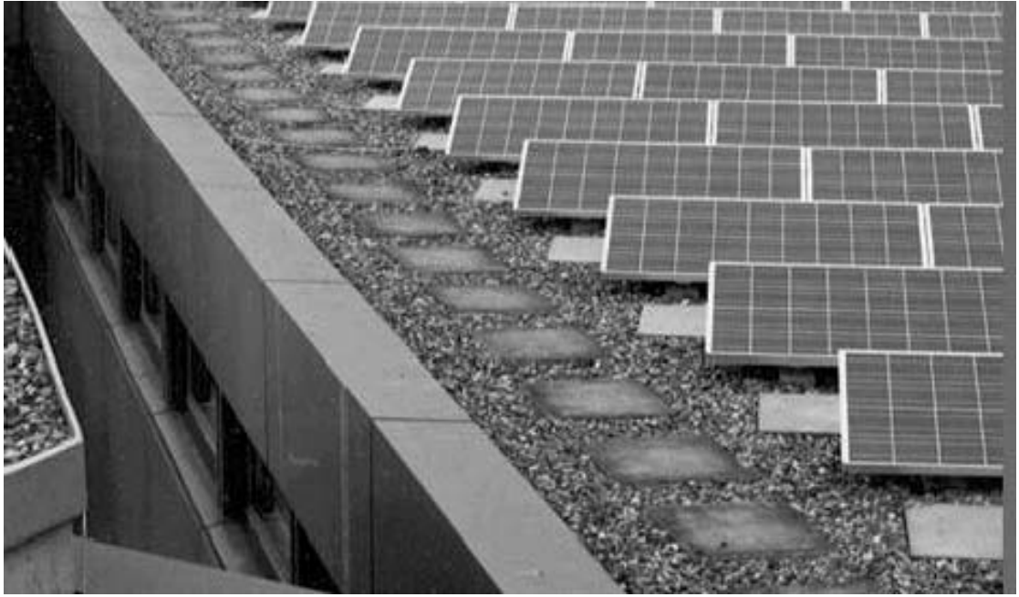
Office building in Wattwil (Switzerland), 30 kW, 1996 built by Tritec (Allschwil, Switzerland) with Sofrel 95-20o and Kyocera modules
