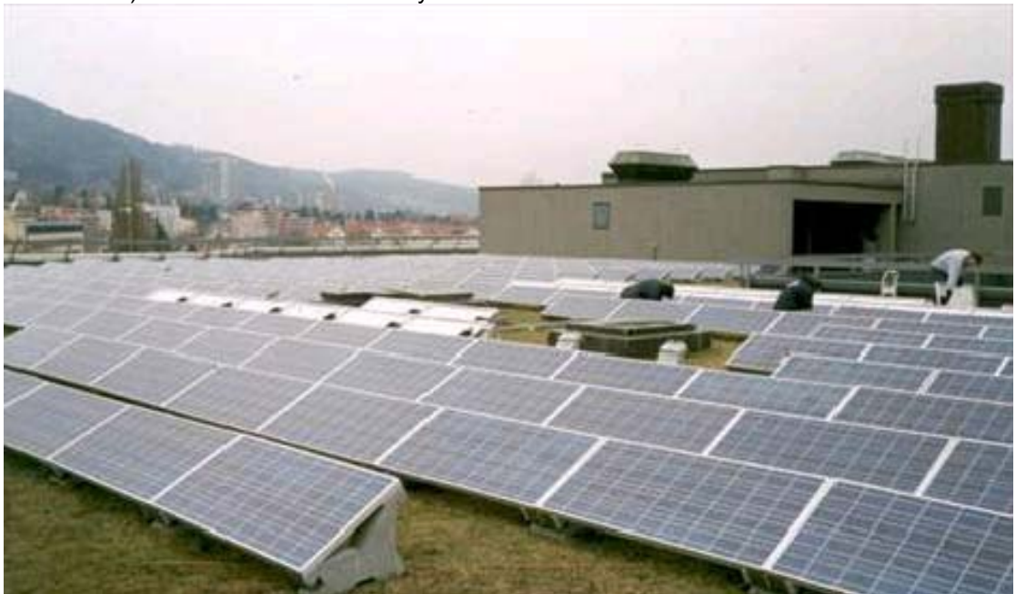
Office building in Wattwil (Switzerland), 30 kW, 1996 built by Tritec (Allschwil, Switzerland) with Sofrel 95-20o and Kyocera modules
