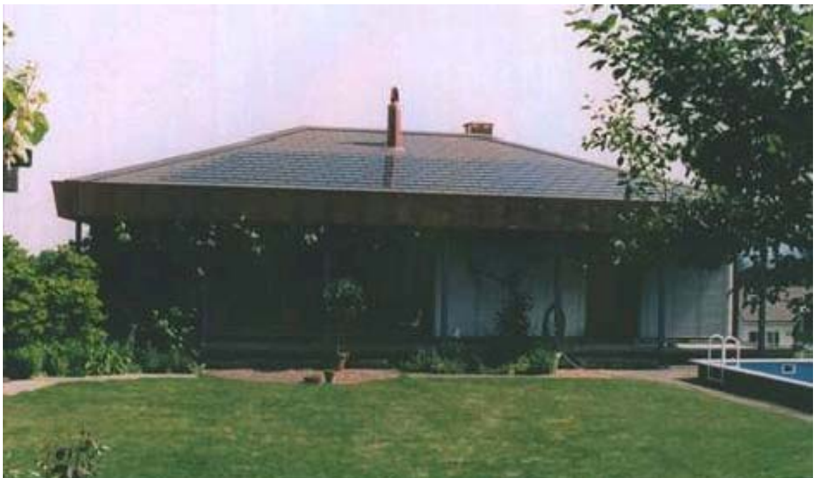
Photovoltaic roof in Aesch (Switzerland), 2.9 kW, 1998, built by Atlantis Solar Systems (Bern, Switzerland)
