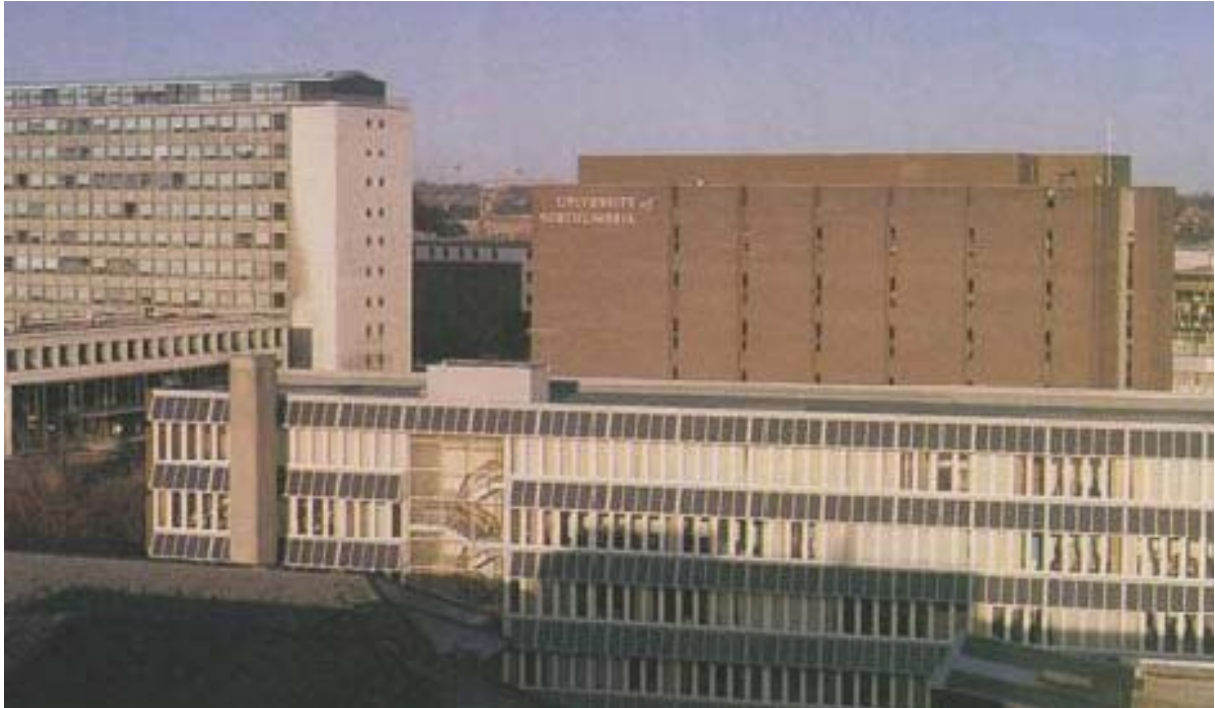
PV facade of the Northumberland Building, University of Northumbria, England, 40 kW, 1994
