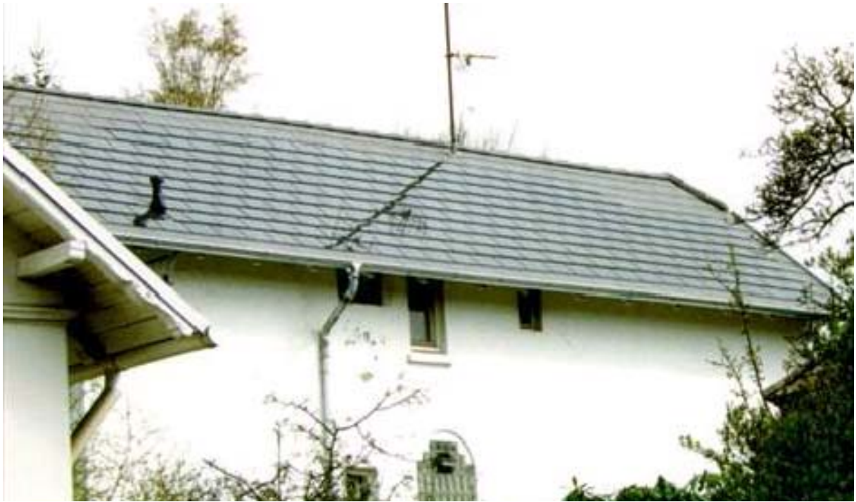
Photovoltaic roof in Hamburg (Germany), 3.4 kW, 1997, built by Atlantis Solar Systems (Bern, Switzerland)
