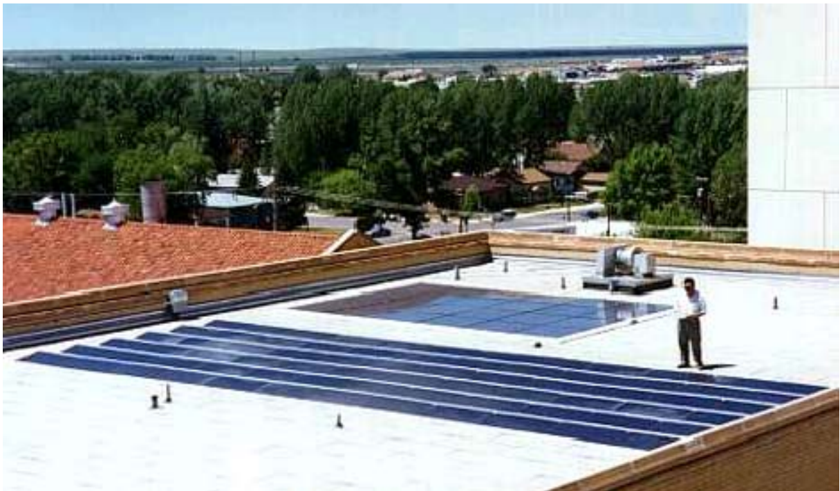
University of Wyoming at Lamarie, USA, 10 kWp includes both sloped and flat tiles, 1996, built by Powerlight
