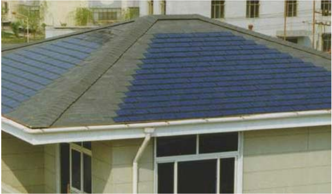
Photovoltaic roof on a house in Beijing (China), 7.5 kW, 1998, built by Atlantis Solar Systems (Bern, Switzerland)
