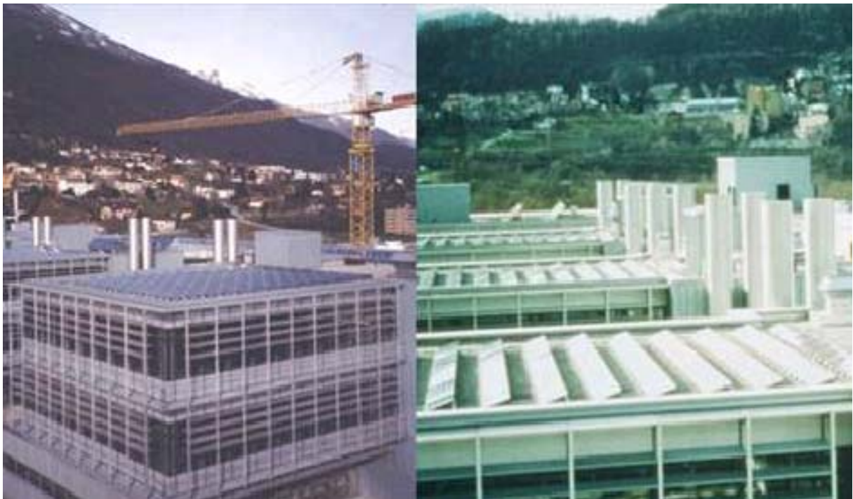
Bank office building in Suglio (Switzerland), 100 kW, 1996, built by Holinger (Liestal, Switzerland) with Sofrel 95-20o and BP modules
