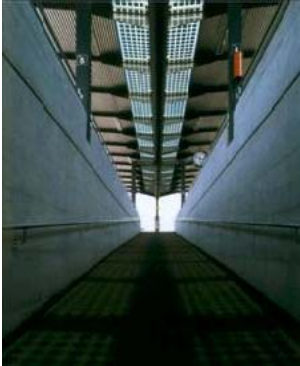
Canopy at the railway station in Morges (Switzerland), 20 kW, 1996, built by Solution (Härkingen, Switzerland)
