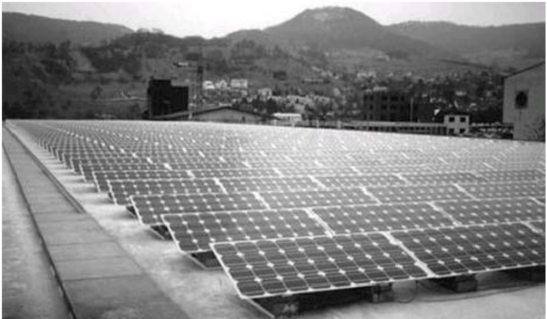
Industrial hall in Sissach (Switzerland), 40 kW, 1996 built by Holinger (Liestal, Switzerland) with Sofrel 95-20o and BP modules
