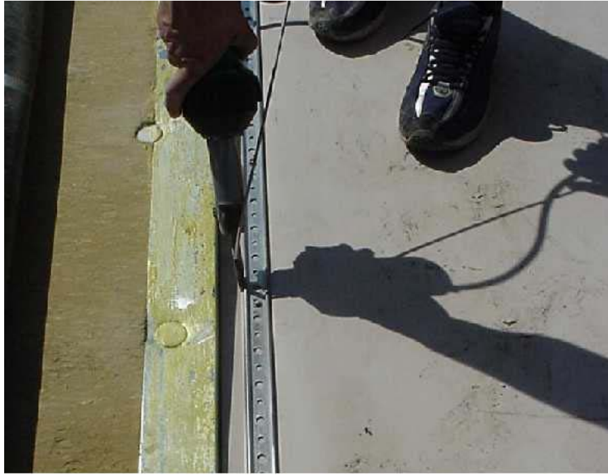
Figure 3: Fixing system to roof.
