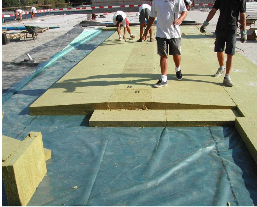
Figure 4: Thermal insulation with 3° tilt for modules support.
