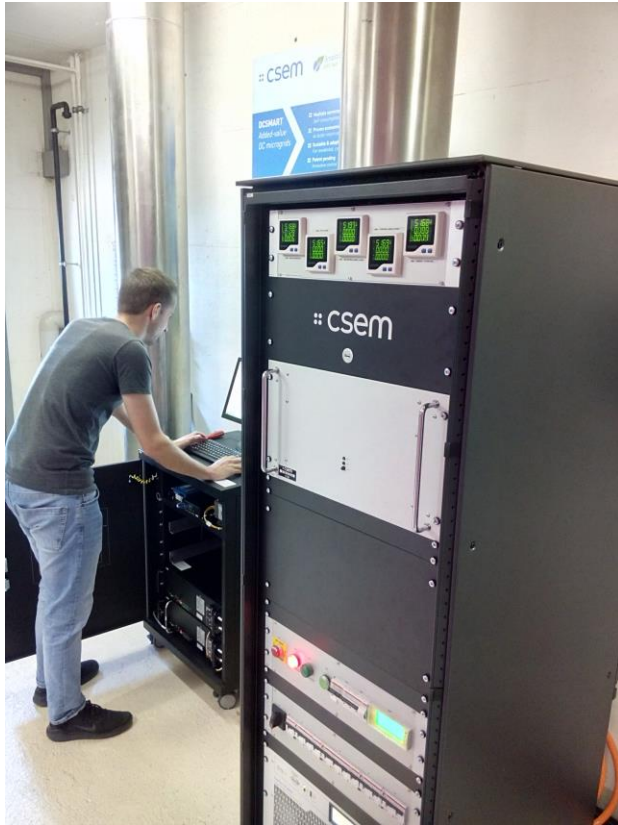
Figure 16: Battery storage cabinet (left) and main electrical cabinet (right) of the demonstrator in operation on the Swiss demonstration site.
