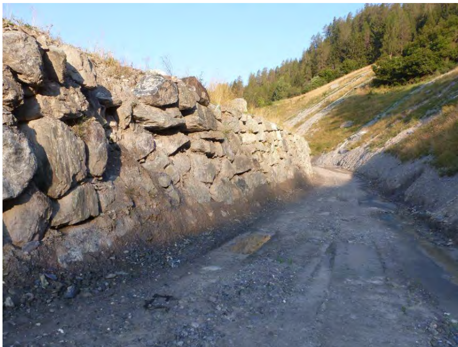
Figure 11 Damage of a RPE with rockery at the uphill side after block impact (Tiefbauamt Graubünden)
