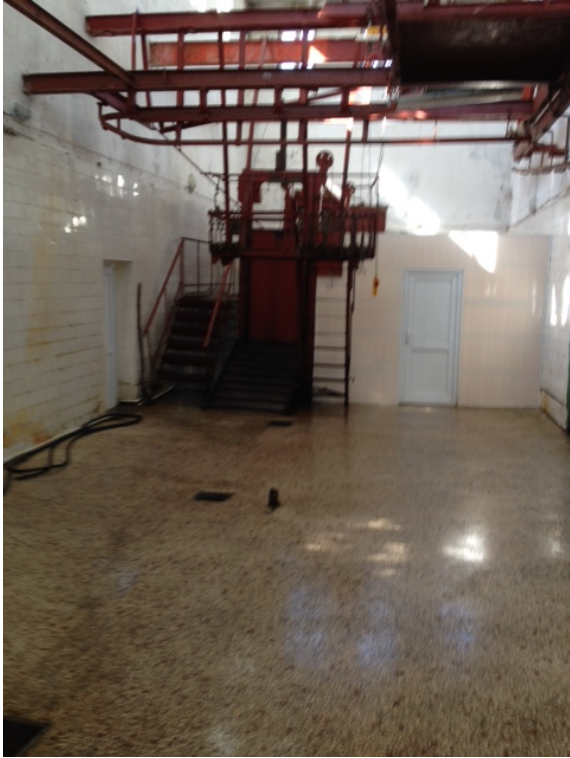
The installation of the slaughter-line for cattle in Ninigori
