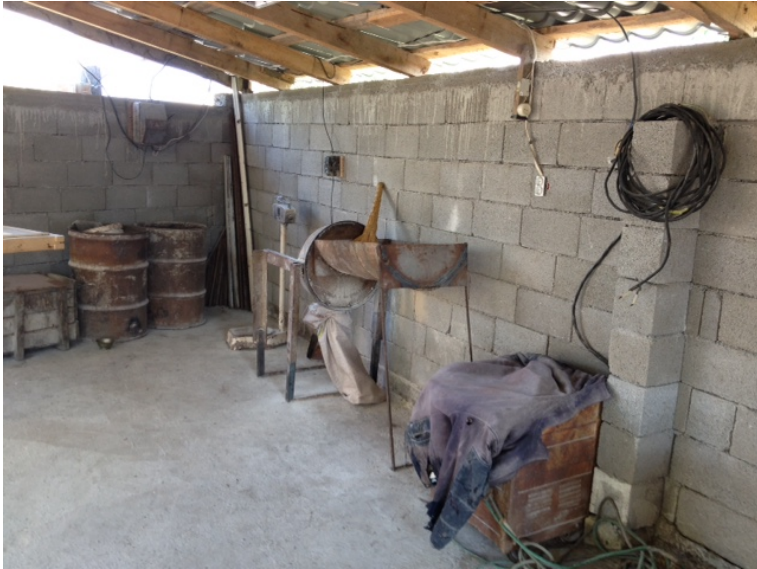
Small mill in Nathisqvilari before up-grading
