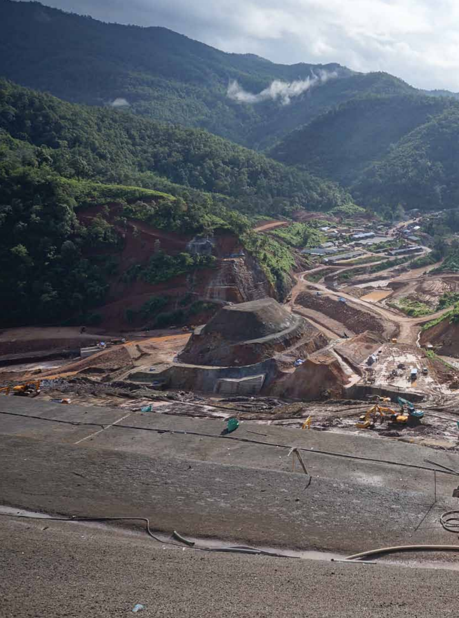
Lignite Mine, Hongsa District, Sayabury Province
