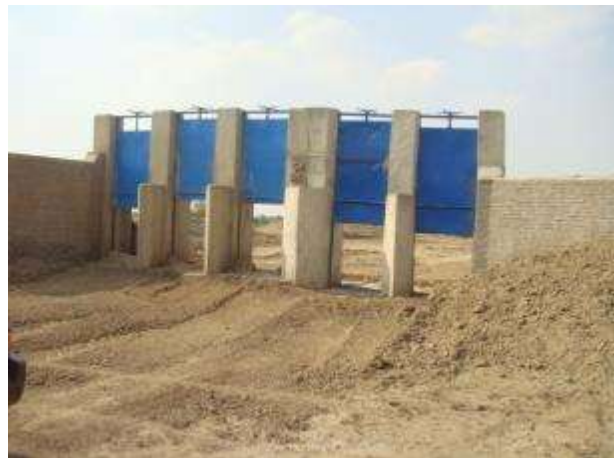
Gate structure supported by W4L in D.I.Khan (photo: Karim Nawaz)
