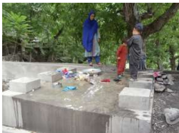
Box 2: Washing pad on irrigation canals in Chitral (photo: Durre Shawar)
