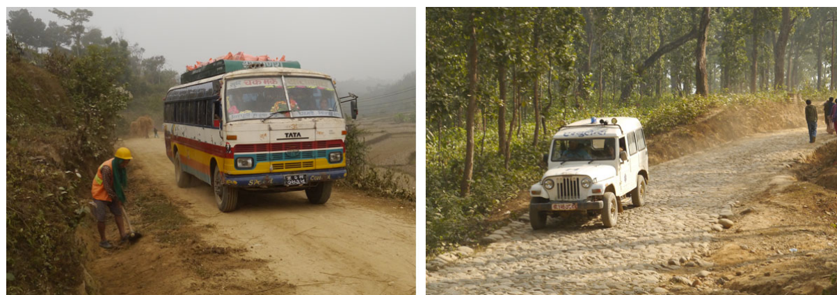
Figure 21: Sections of Sindhulimadi-Bhimsthan road with length person, bus, ambulance and cobblestones
