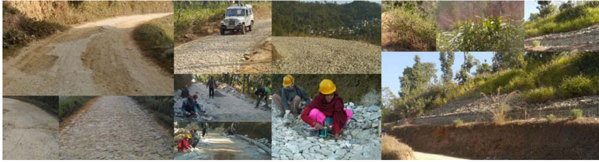
Figure 11: Montage of DRSP activities relating to pavement trials, cobblestones and bioengineering
