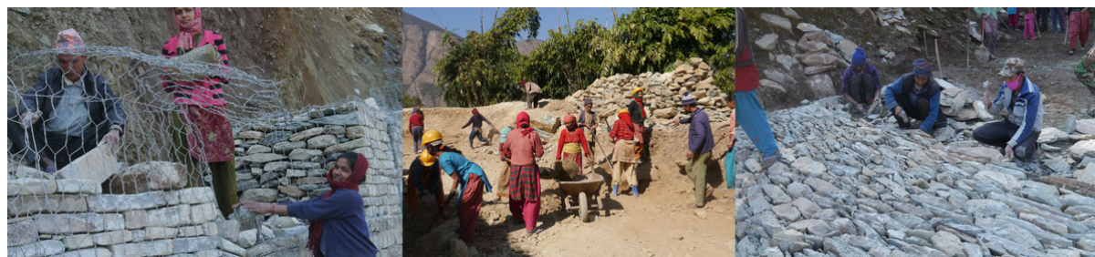
Figure 10: Labour-based construction provides labouring and skilled employment
