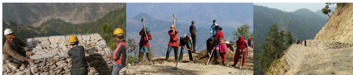
Figure 23: Construction on the Khimti-Betali-Namadi road
