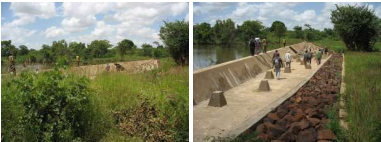
Newly constructed dam in Koba village
