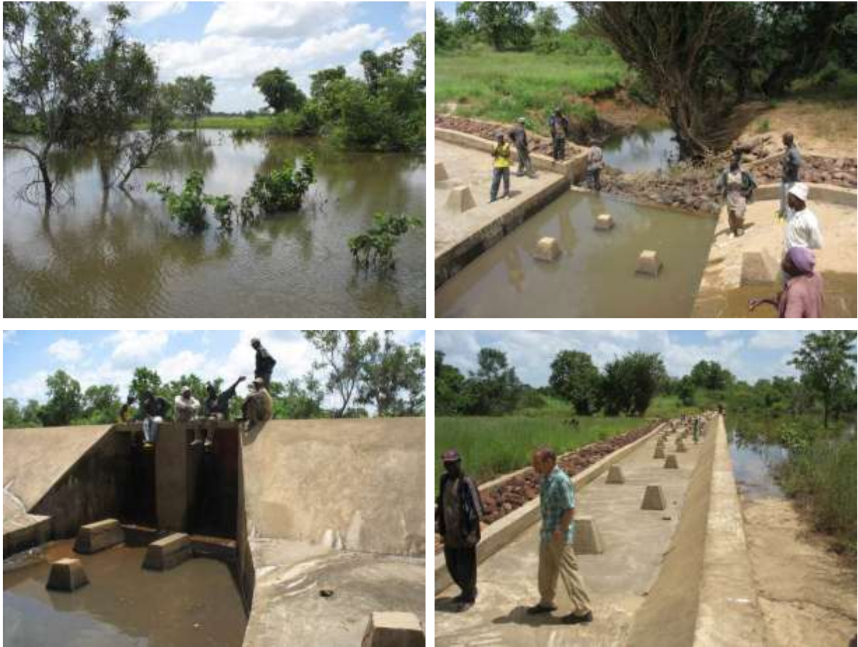
Newly constructed dam in Koba village
