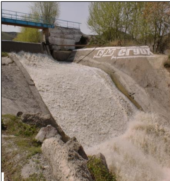
Aksu River flowing through Canal in Spitamen without gate
