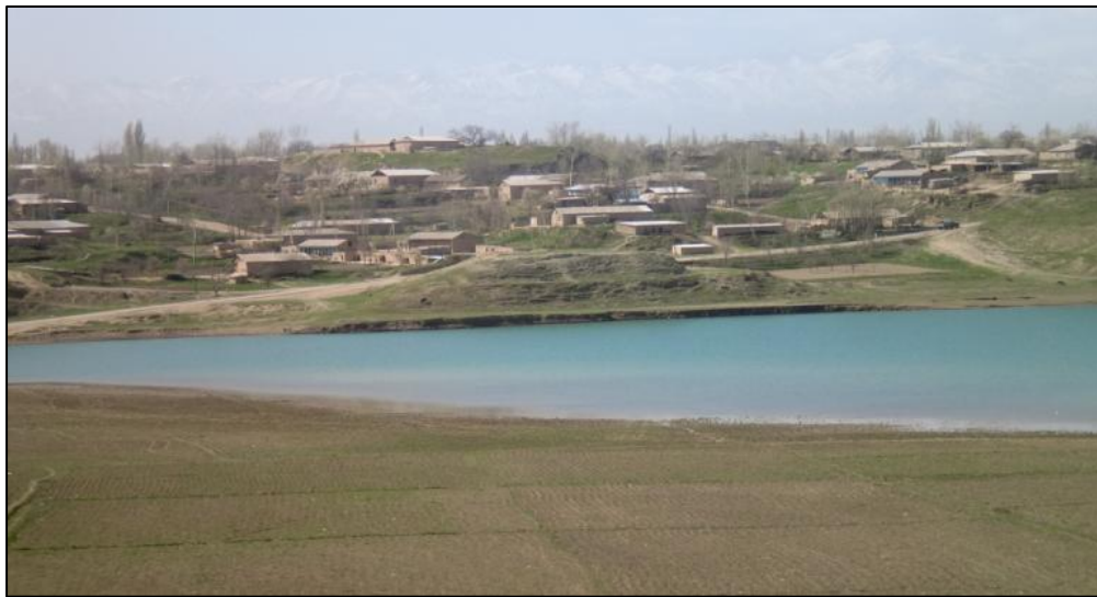
Dahanasoy Water Reservoir – Ghonchi District
