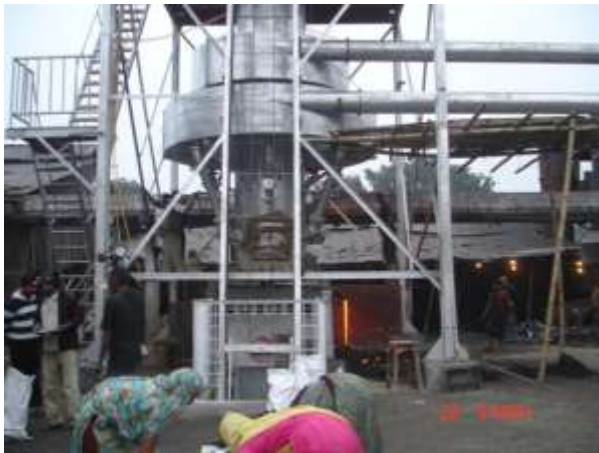
Bucket charging system
