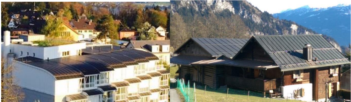
Figure 1: Examples of metal roof tops in Switzerland ready for Flisom solar modules
