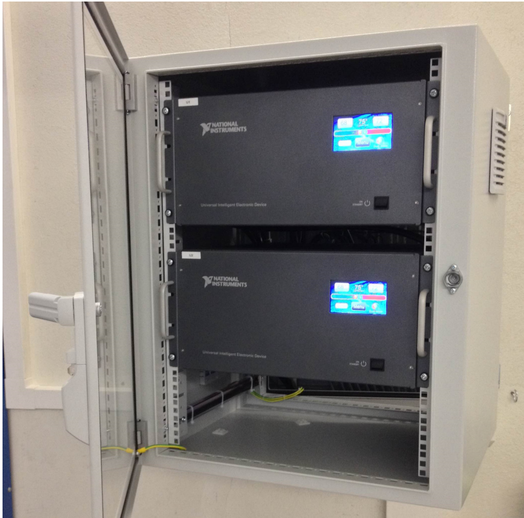
Figure 3 - PMU installation in an electrical substation of the 125-kV grid of Lausanne.
