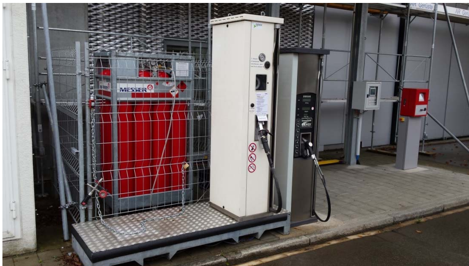
Fig. 3.1: Ad interim solution for refueling CNG with slight hydrogen addition (2 vol%)
