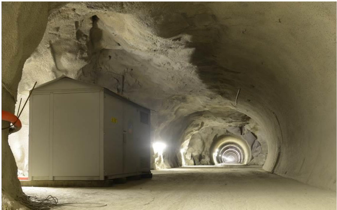
Fig. 6: The 600 kW oil-free transformer supplied by AET.
