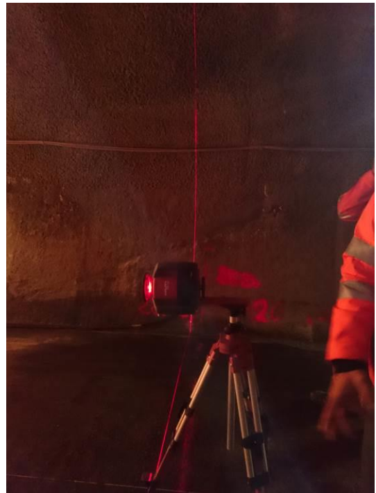
Fig. 7: Left: Cutting the tunnel floor to subsequently dig and place the necessary tubes (water, current, signals). Right: Marking the exact position of the plugs using laser markers.
