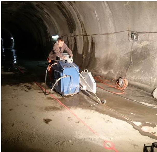
Fig. 7: Left: Cutting the tunnel floor to subsequently dig and place the necessary tubes (water, current, signals). Right: Marking the exact position of the plugs using laser markers.
