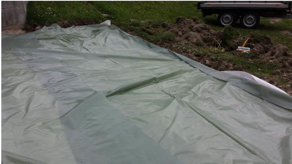
Fig. 4: Fluid capturing membranes placed at the Loderio side of the tunnel. The membranes are later covered with approx. 20 cm of soil.
