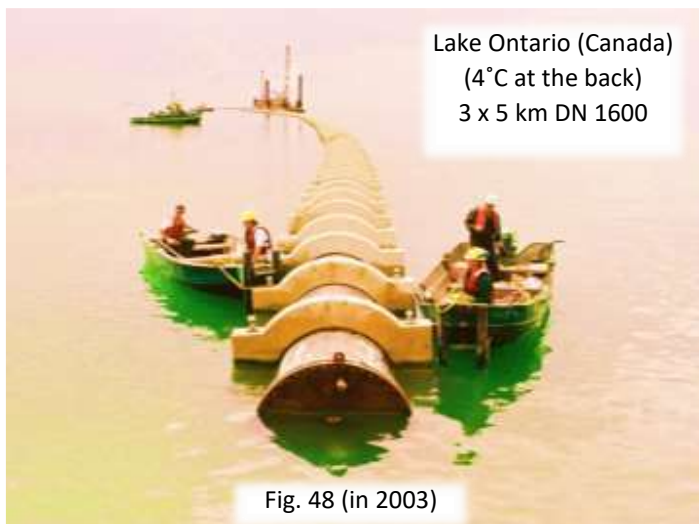
Fig. 50 Transport (Lake Ontario) of the HDPE pipe ( \varnothing 1.6 m x 15 km!) for pumping and supplying water of the Deep Lake Water Cooling (DLWC) system in the Canadian city of Toronto (Enwave image)
