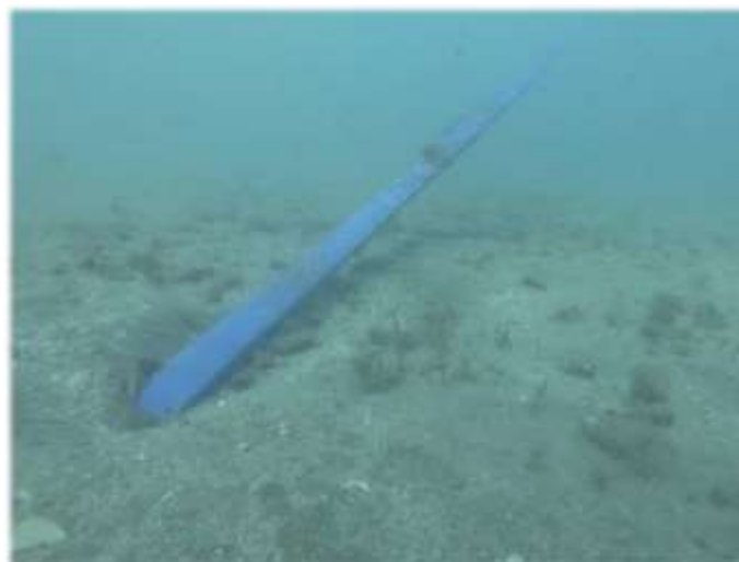
Fig. 55: Impact of a helical anchor aimed at the lake bed (Screw-in Anchor Technology, marinflex.com)
