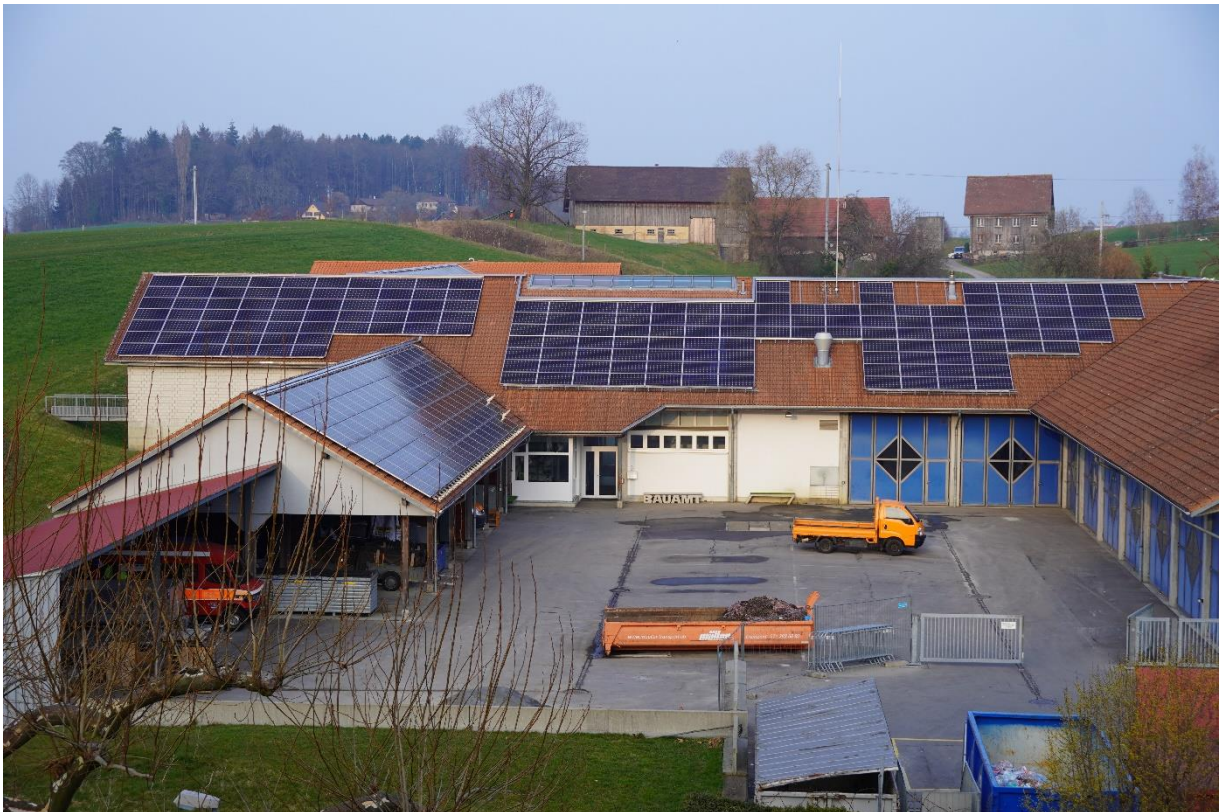
Source: ©Nicolas Stocker 2023 (Werkhof (work yard), municipality Wittenbach)
