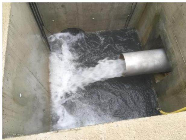
Figure 9: Wellhead of G<sub>Eo</sub>-1 producing thermal water containing a black-coloured suspended load.
