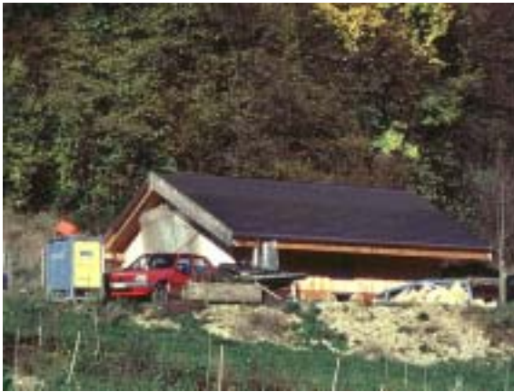
Figure 20: Stand-alone 3 kWp roof integration in Soyhières (Photo: NET)
