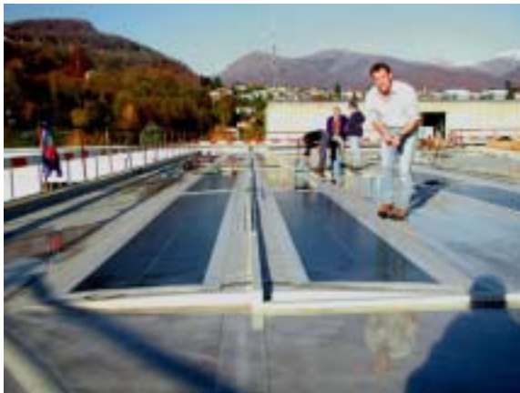
Figure 18: Construction of the CPT Solar Trevano (Photo: LEEE-TISO)
