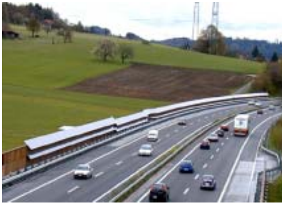
Figure 34: 75 kWp noise barrier installation A1 Safenwil (Photo: BFE)
