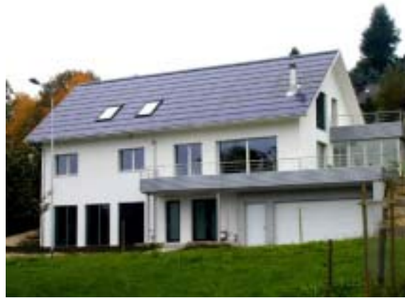
Figure 13: Erni' solar house with SOLRIF roof integration (Photo: Enecolo)
