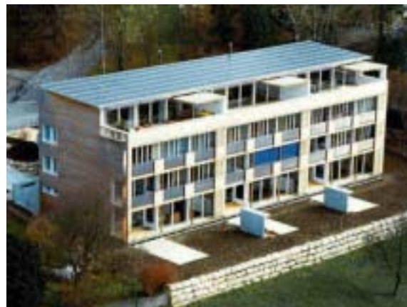
Figure 15: Sunny Woods 16 KWp roof integration (Photo: Beat Kämpfen Architectural Consultants)
