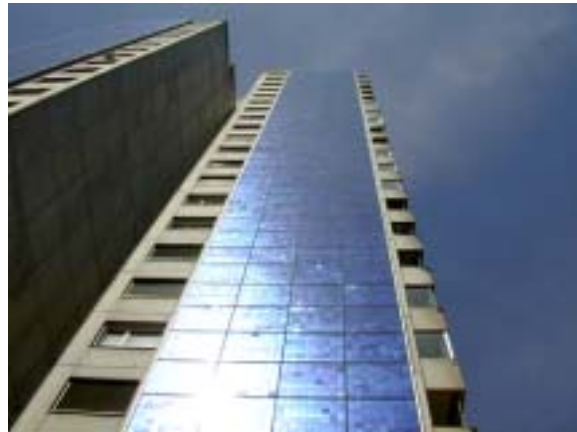
Figure 21: 80 kWp facade in Wittigkofen near Bern (Photo: NET)
