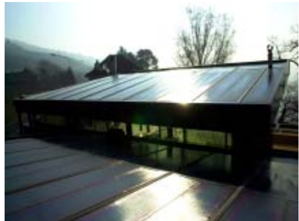
Figure 25: Freestyle® roof integration in Lutry (Photo: Solstis)
