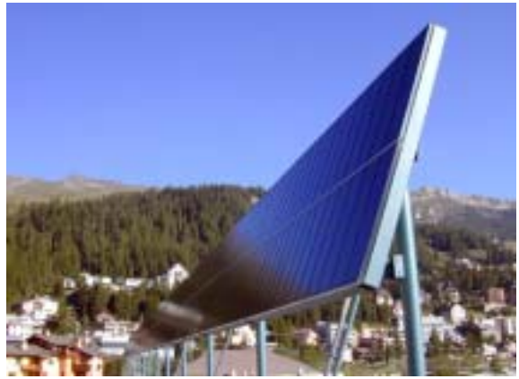
Figure 35: 16.8 kWp installation with CIS cells in St. Moritz (Photo: NET)
