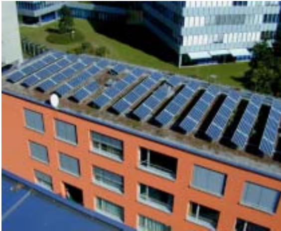
Figure 28: Solgreen Kraftwerk 1 green roof installation (Photo: NET)
