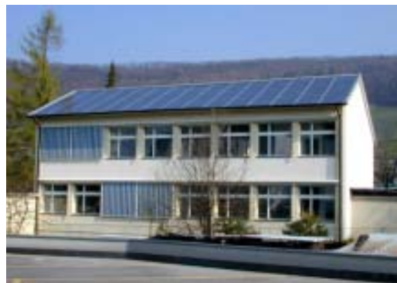
Figure 31: 12.75 kWp roof integration in Wettingen (Photo: NET)
