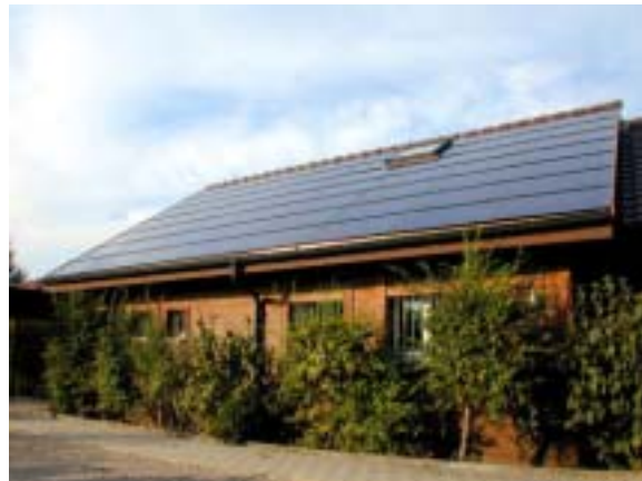
Figure 19: Pfadiheim Weiermatt roof integration installation in Köniz (Photo: NET)
