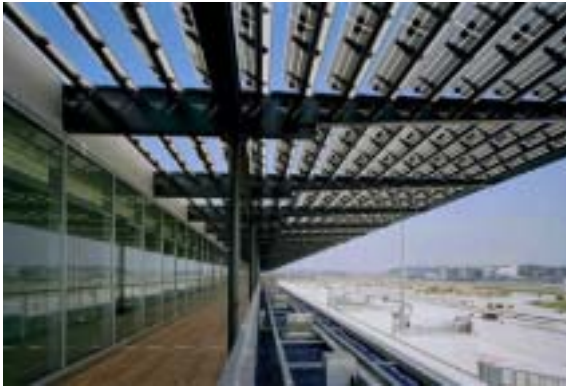
Figure 16: Dock Midfield PV shading installation (Photo: unique / Ralph Bensberg)
