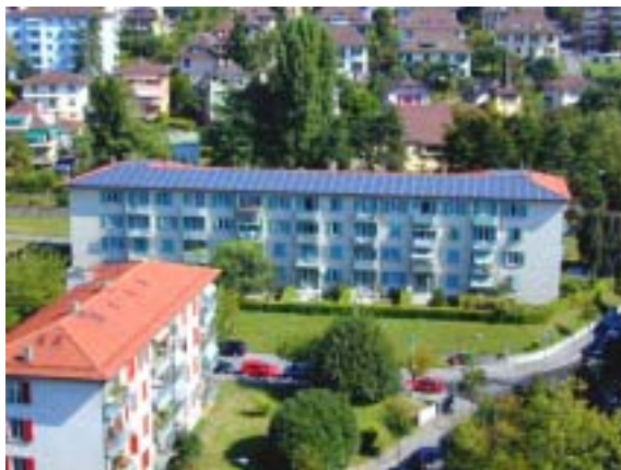
Figure 14: Florency SOLRIF roof integration in Lausanne (Photo: NET)
