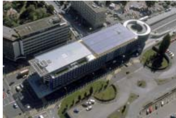
Figure 17: Parking de l'Etoile roof integration in Geneva (Photo: Sunwatt Bio Energie)
