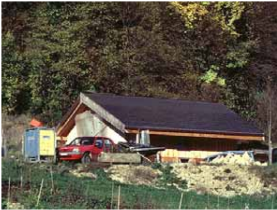
Figur 20: Autonome 3 kWp Dachintegration in Soyhières (Bildquelle NET)
