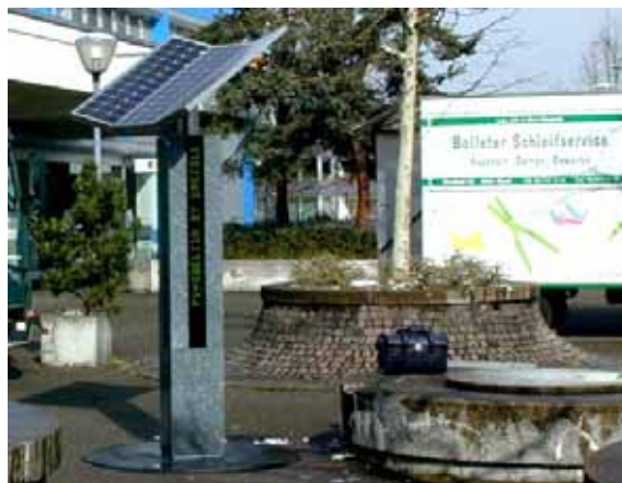
Figur 27: Autonomer Photovoltaik Obelisk Zürich (Bildquelle Enecolo)
