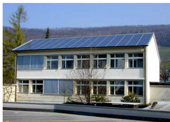
Figur 31: 12.75 kWp Dachintegration Wettingen (Bildquelle NET)
