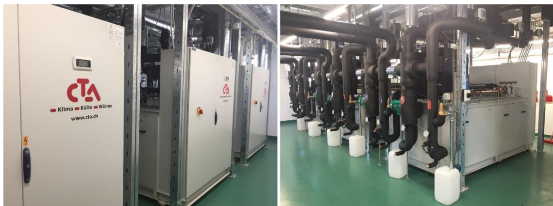
Figure 15: The three tailor-made water/water CTA heat pumps (Type: PC-42.604-W.W-1234ze-HT-LN). The machine room offers space for up to 8 machines with a final cooling capacity of 2 MW.
