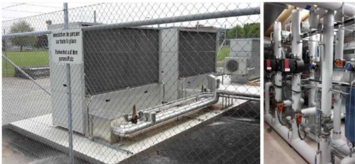
Figure 47: CO 2 heat pump from ENEX and heat distribution for the Swiss Army Training Hall in Payerne [43].
