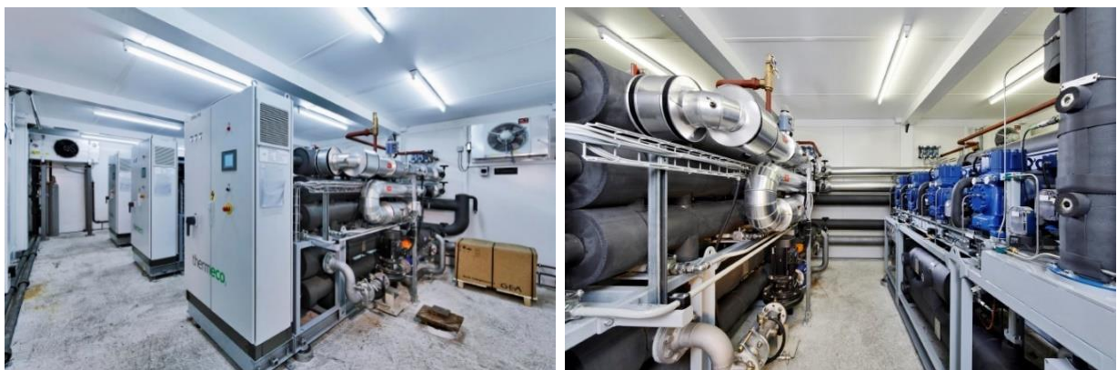
Figure 40: Three CO 2 heat pumps of the type thermeco 2 HHR 260 at the slaughterhouse in Zurich [35,37]
