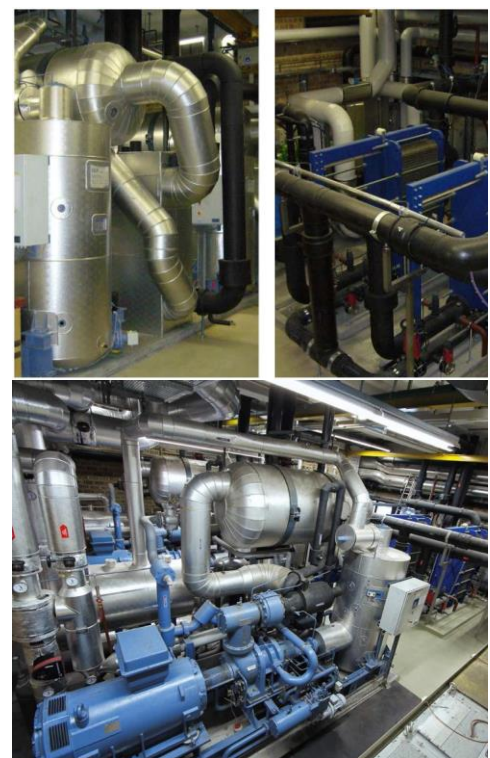
Figure 42: Front view of the two heat pumps and plate heat exchangers for waste water with filter systems [38], [39].
