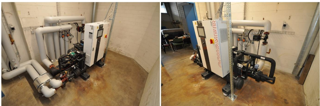
Figure 10: Ochsner heat pump (Type: ISWHS 60 ER 3, economizer cycle) in the heat center of the agricultural cooperative association Schaffhausen (GVS) (Photos from ennovatis Schweiz AG).
