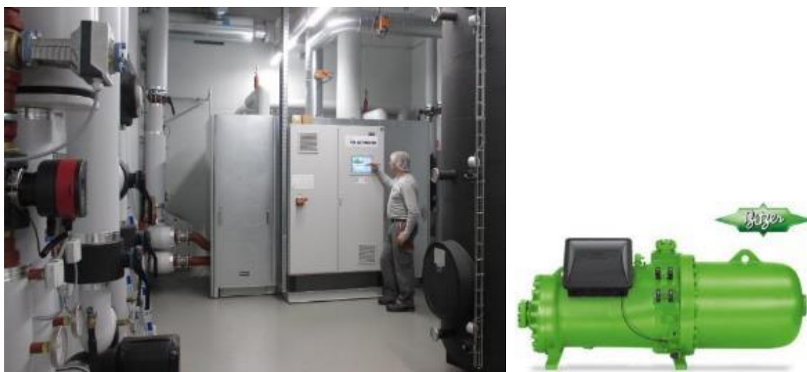
Figure 57: Heat pump from Friotherm AG (Type X22HE-450A) running with screw compressor from Bitzer (CSH9573-180Y) and HFO refrigerant R1234ze.
