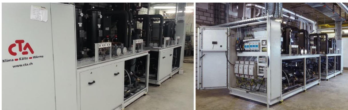
Figure 23: Two CTA exklusiv air/water heat pumps with up to 265 kW heating capacity each. The installation provides accessibility for maintenance and service [22,23].
