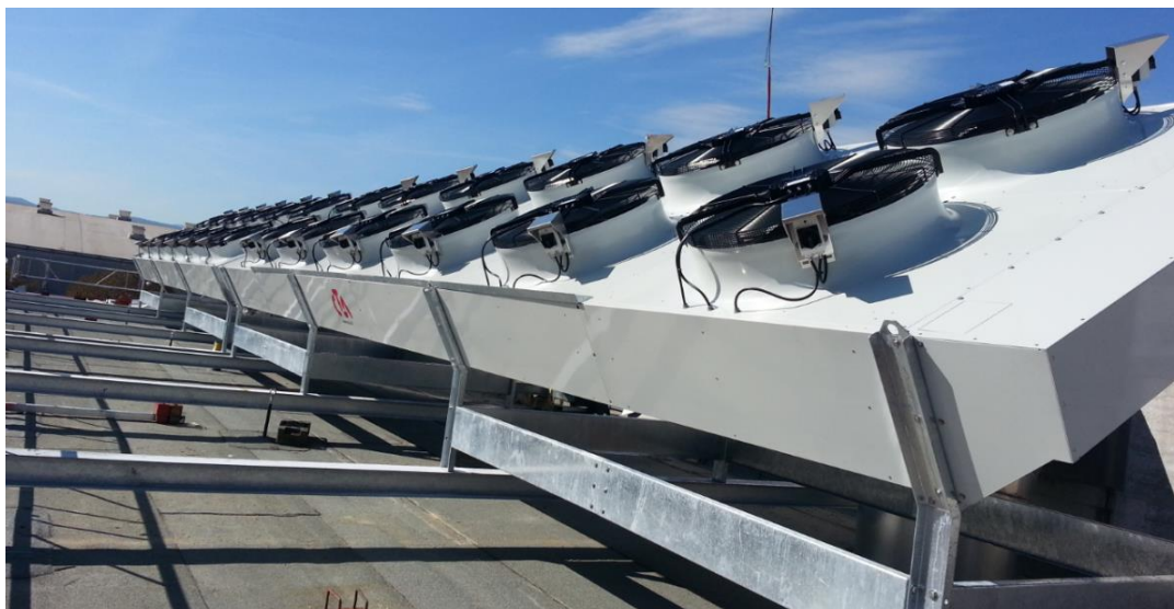
Figure 24: One of the two 11 m long air coolers, which extract the source energy from the air [22].
