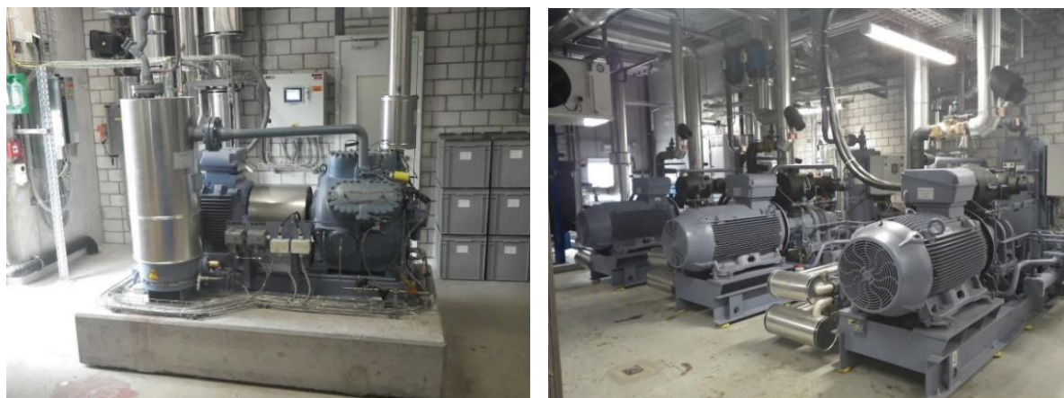
Figure 60: Left: GEA Grasso 65HP with 6 cylinders and oil separator for waste heat recovery. Right: GEA Grasso RB-5A chillers with screw compressor at Hilcona AG in Schaan (FL).
