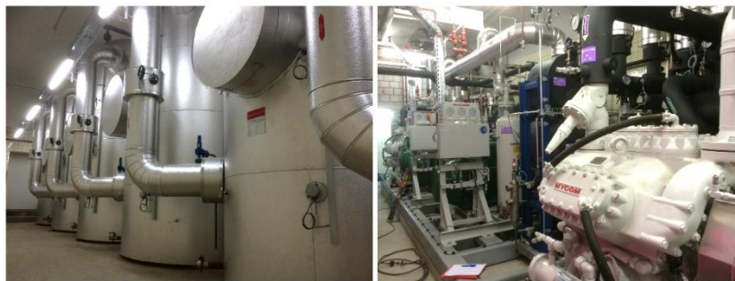
Figure 55: Storage tanks (3 x 58 m 3 ) for the waste heat and Mayekawa MYCOM compressor [54].
