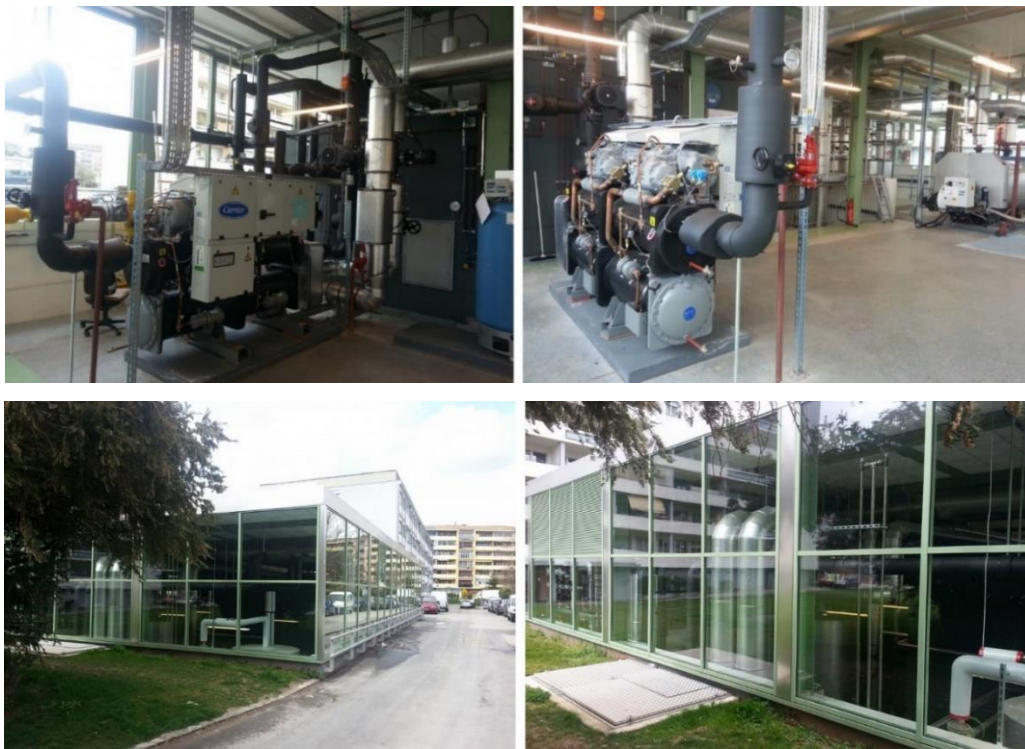
Figure 62: Central heating center at Laurana-Parc with the installed heat pump from Carrier (30HXC 080 - option 150 high temperature version). The heat pump uses R134a and runs with a screw compressor. The nominal heating capacity is 338 kW at 14-16/8 °C heat source and 58/63 °C sink temperature with a COP of 3.45 [58] (Photos from Conti & Associés Ingénieurs S.A. [59]).
