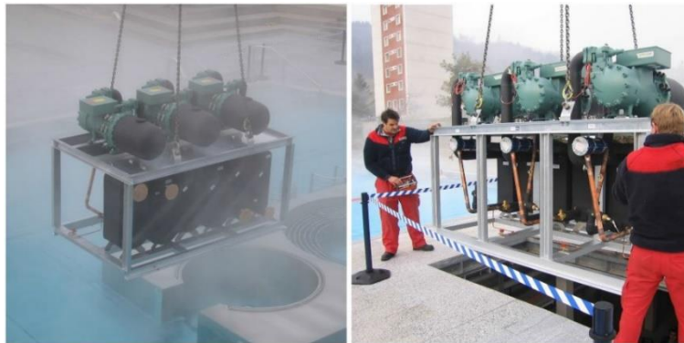
Figure 39: Installation of the new water/water heat pump for heat recovery of waste thermal water with two special cranes in the area of the thermal bath [33].
