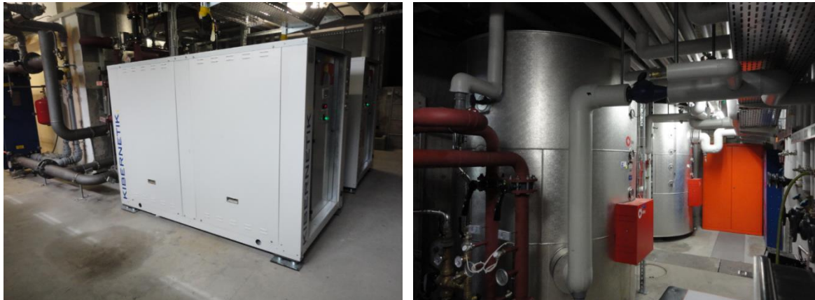
Figure 31: The two groundwater heat pumps from Kibernetik AG and the hot water storage tank installed at the Swiss army troop accommodation building in Matt.
