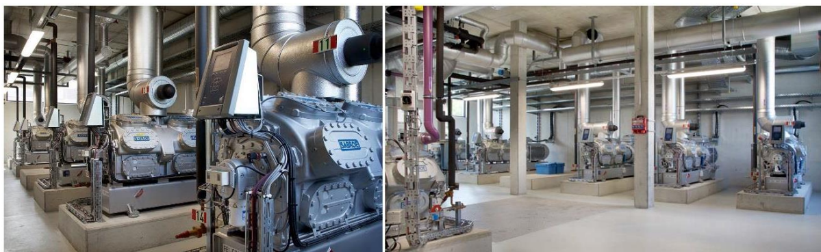
Figure 51: The installed NH 3 compressors (Sabroe, Johnson Controls) in the energy center of Mifa AG at Frankendorf. Three compressors (JC/Sabroe SMC 116 LV) for the -29°C cold, two compressors (JC/Sabroe SMC 112 LV) for the ice water production with 2°C, and one heat pump (JC/Sabroe HPC 106 SV) for heat recovery providing 70 °C [47,48].
