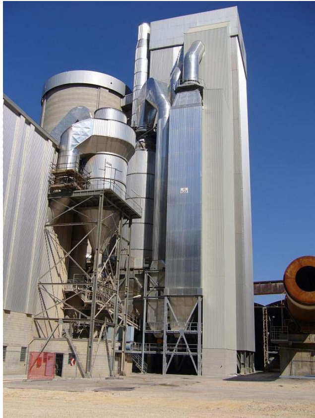
Figure 1. SCR reactor at Cementeria di Monselice
