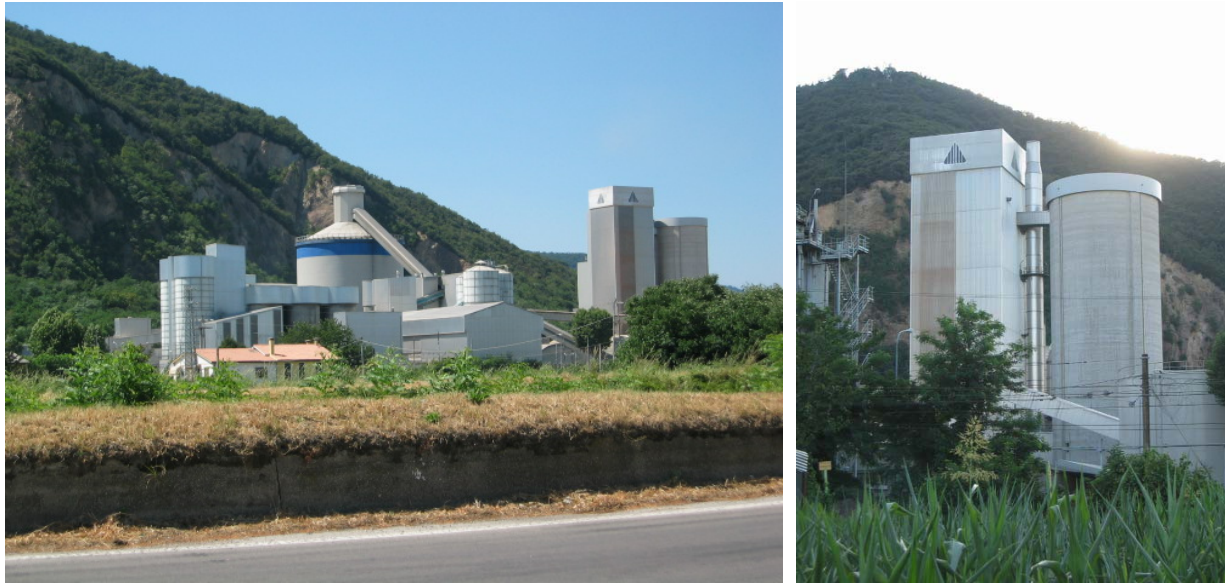
Figure 3. Photograph of Cementeria di Monselice from East. Preheater Tower, Feed Silo, Stack
