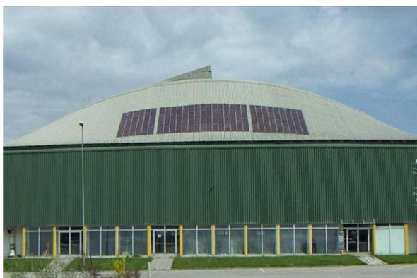
**Figure 11:** Toiture Flexcell expérimentale de 2 kW<sub>c</sub> (Source: VHF-Technologies)
