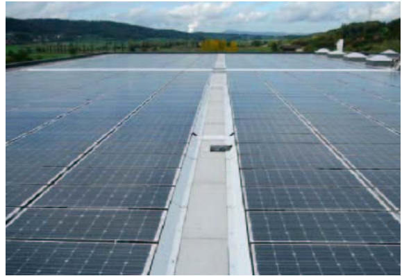
Figure 11: 62 kWp flat roof installation with Power Guard solar roof panels (Photo: Zagsolar)
