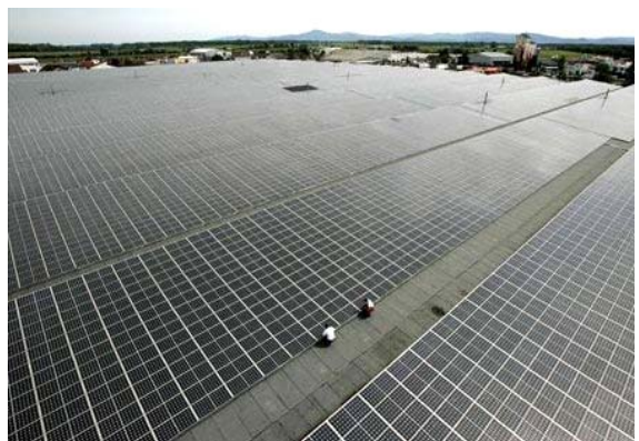
Figure 7: 5 MWp Sonnenfleck roof integration ( www.sonnenfleck.com )
