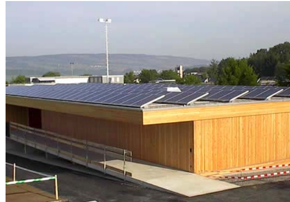
Figure 5: Hünenberg 27 kWp Alustand installation (Photo: Urs Bühler Energy Systems)
