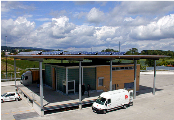
Figure 10: PV installation on Kreuzlingen Zollhof (customs building) (Photo: NET)
