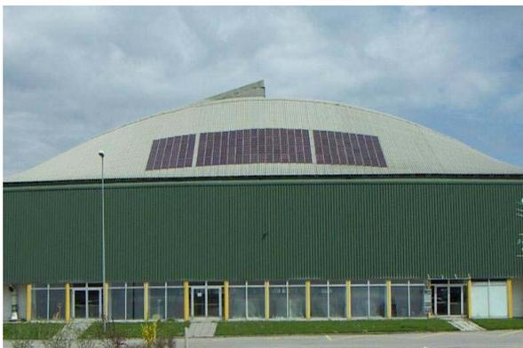
**Figur 11:** 2 kWp Flexcell Experimentaldach
