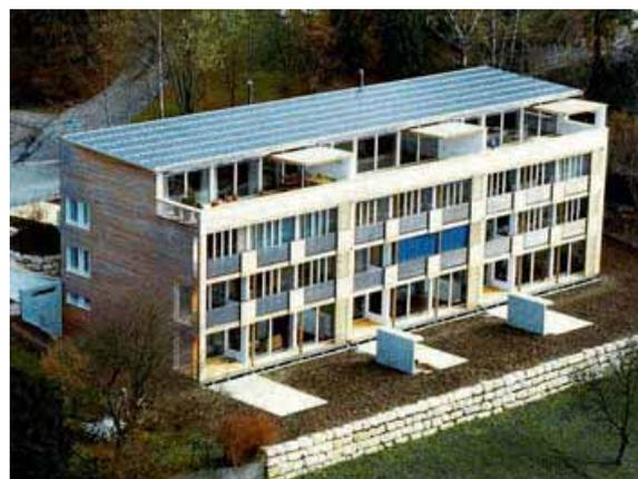
**Figur 15:** 16 kWp Dachintegration SunnyWoods
